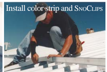
Fasten to structure through pre-punched holes (screws not by S-5!)
