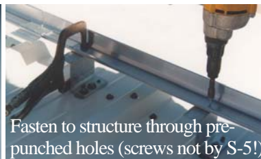
Install color strip and SNOCLIPS
