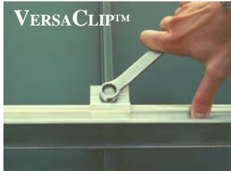
Slide VERSACLIPS into COLORGARD
